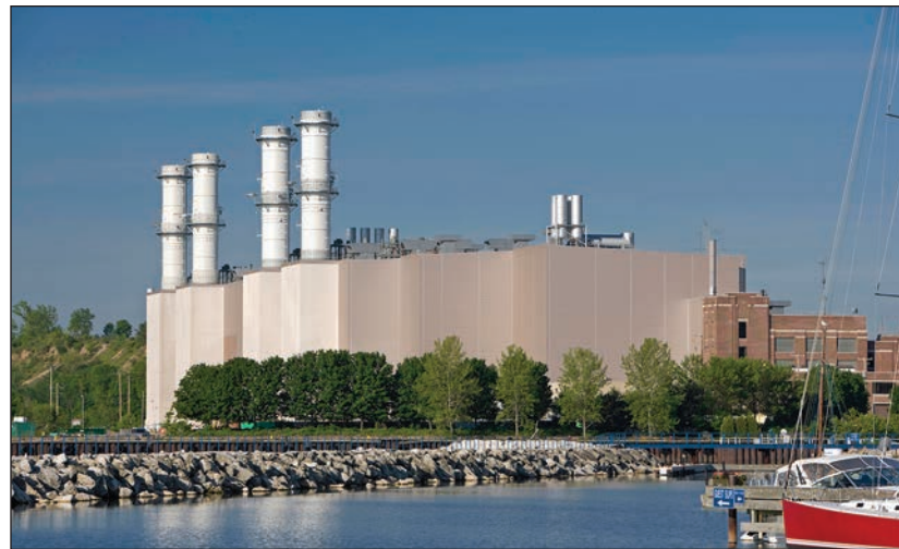
Port Washington Generating Station, Port Washington, Wisconsin
