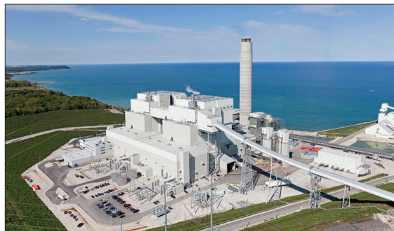
Oak Creek Expansion Units, Oak Creek, Wisconsin
