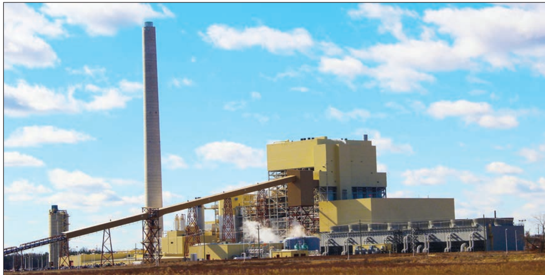
AEP's 600-megawatt John W. Turk Jr. Power Plant in Arkansas began operation in December 2012 and is the first in the United States to use ultra-supercritical advanced coal combustion technology, which requires less coal and produces fewer emissions to generate the same amount of power. (above) Nick Akins interacting with employees at the Turk Plant during the plant's early construction phase. (below)
