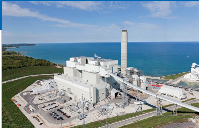
Wisconsin Energy's Oak Creek Expansion Units, Oak Creek, Wisconsin
