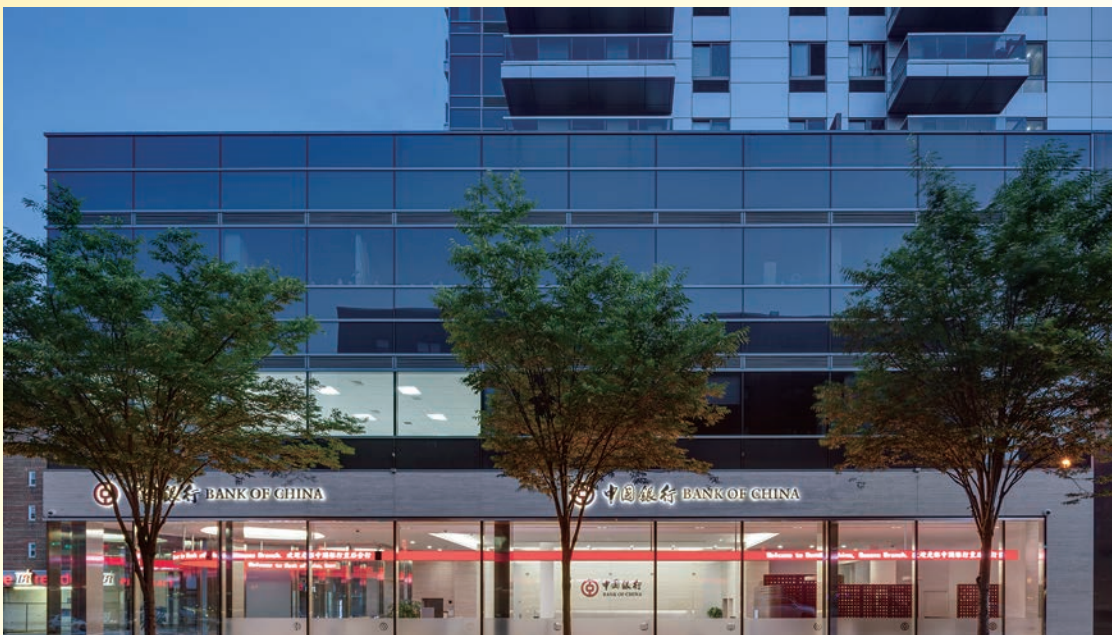
Exterior of the branch in Queens
