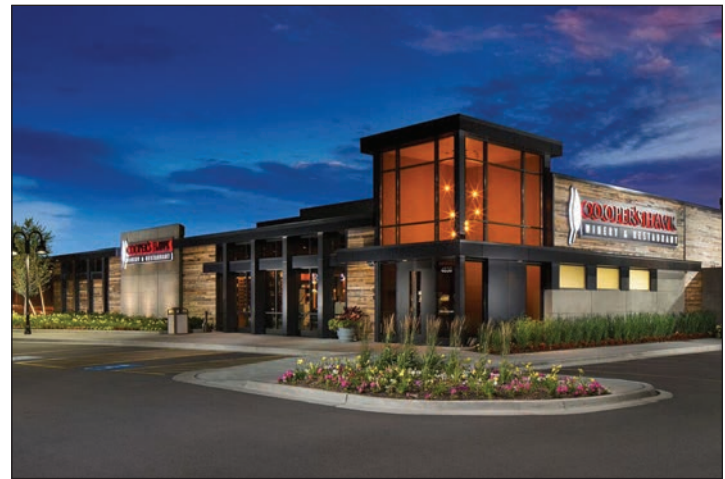
Interior of the Cooper's Hawk on International Drive in Orlando, Florida (left); exterior of the Cooper's Hawk in Oak Lawn, Illinois (above)
