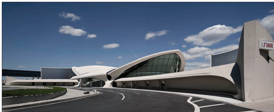
A rendering of the Eero Saarinen-designed TWA terminal that MCR is redeveloping into a hotel (above) Homewood Suites by Hilton in Phoenix-Avondale (below)
