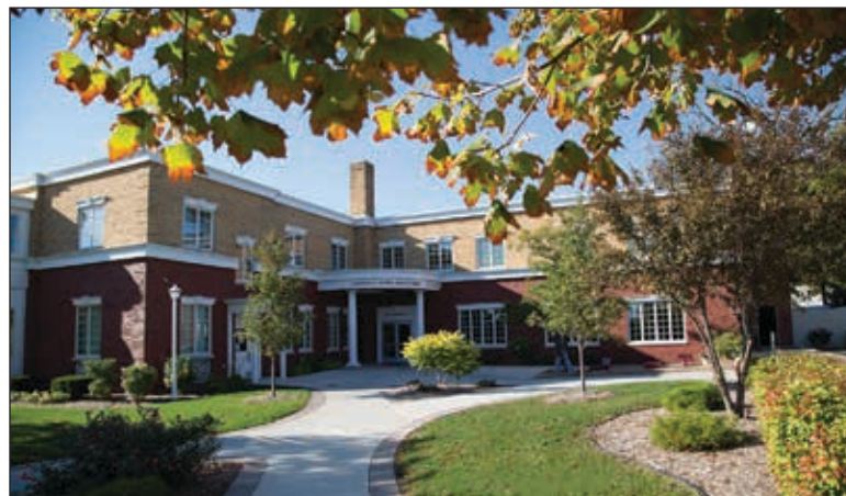
Carriage Town Ministries main building
