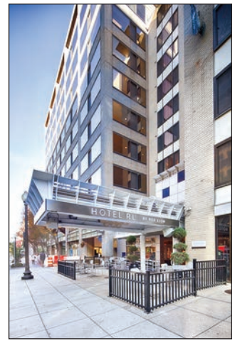
Hotel RL in Washington, D.C. exterior (above) and guestroom (left)
