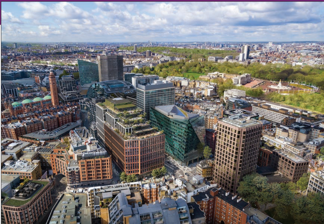
105 Victoria Street, London, BentallGreenOak's ground-breaking development scheme that will deliver London's largest net-zero, 100 percent electric-powered office building
