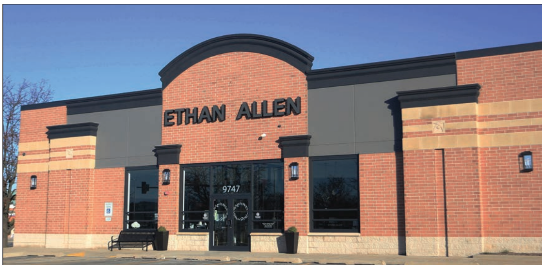
Ethan Allen Design Center in Skokie, Illinois
