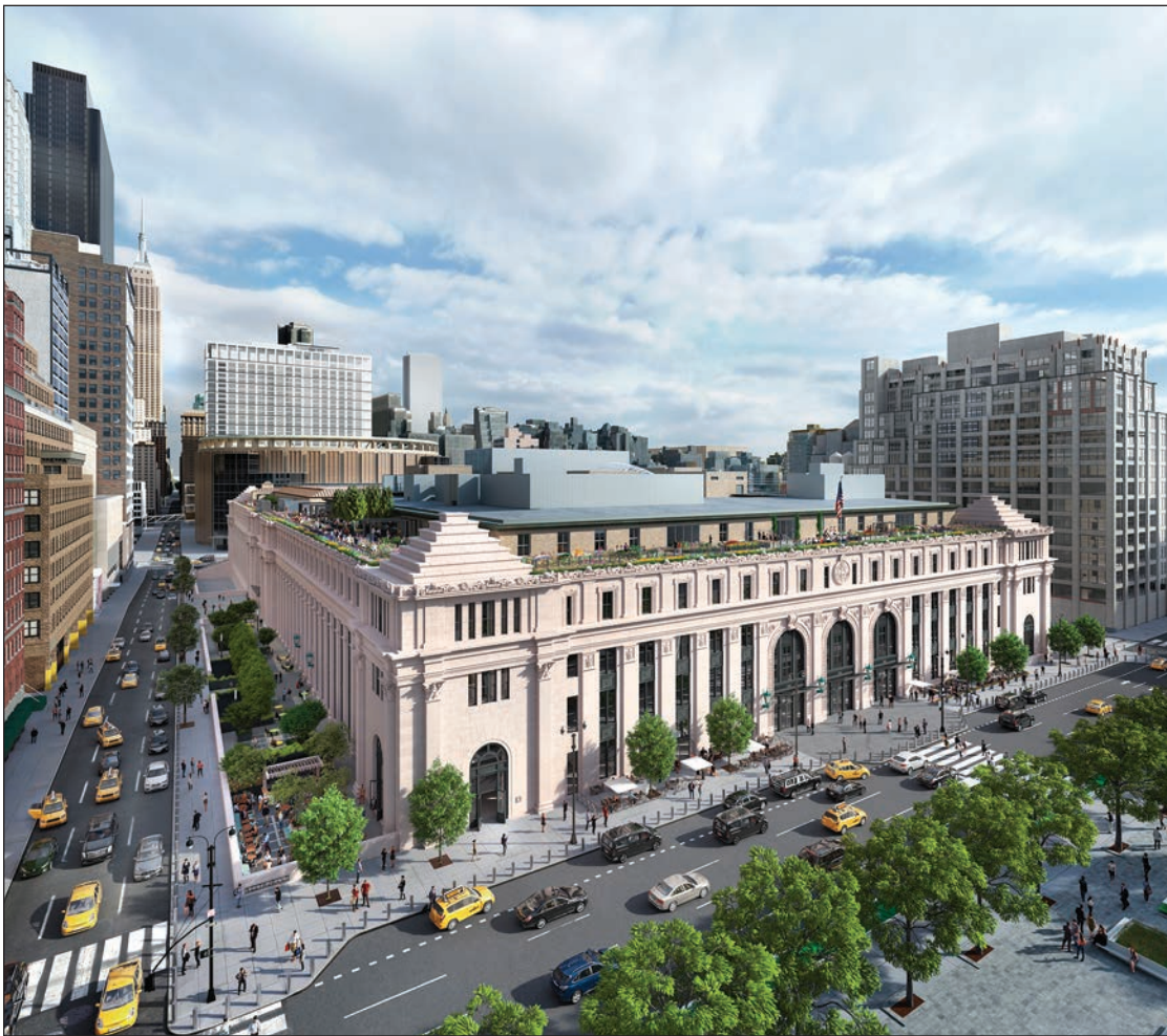
The Farley Building at 390 Ninth Avenue is being transformed by Vornado into a New York City creative office hub
