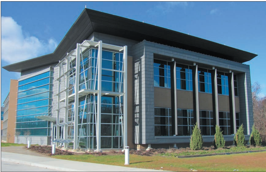
Advanced Energy Research and Technology Center at Stony Brook University
