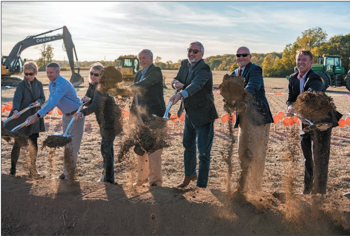
Governor Holcomb breaks ground in Princeton, Indiana for the Toyota Indiana YMCA, a project funded by READI
