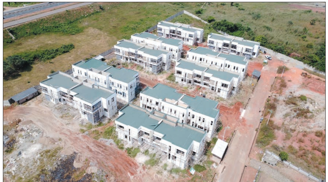
Aerial view of the ongoing 20 unit detached duplex project at the PMB Housing Estate, Abeokuta Ogun State, Nigeria by Still Earth Construction
