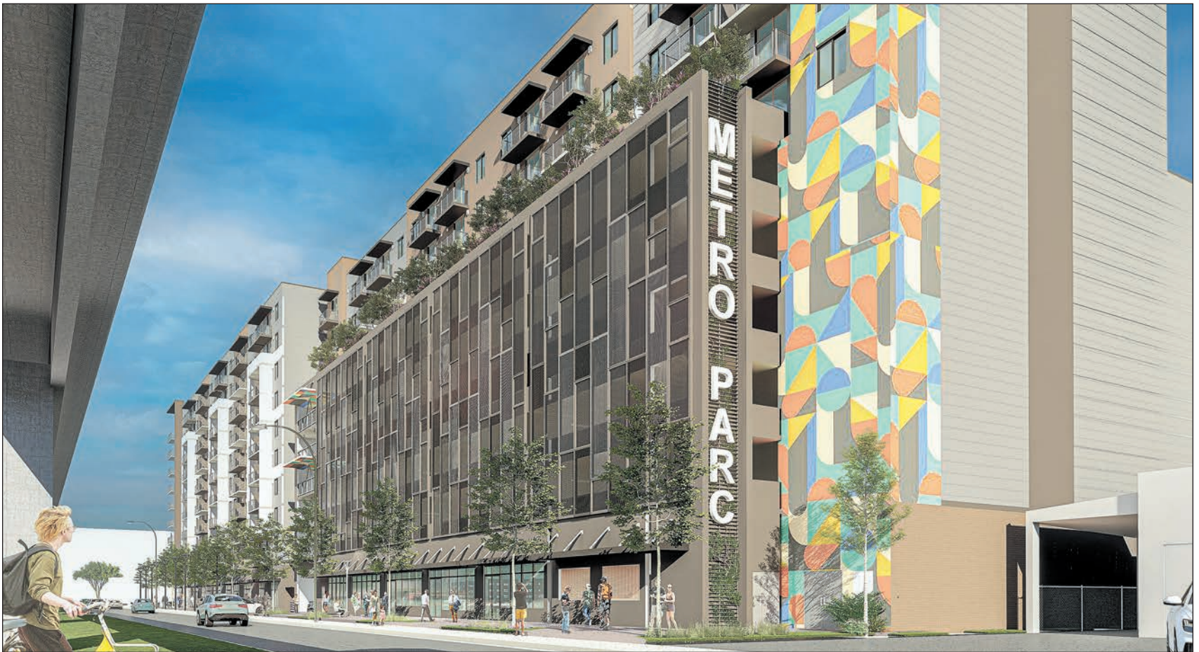
Baron Property Group is currently building Metro Parc, the first phase of its 2.3-million-square-foot mixed-use development in Hialeah, Florida (above); The Park Overture brings well-designed, full-service rental homes and park-side living to Washington Heights (below)
