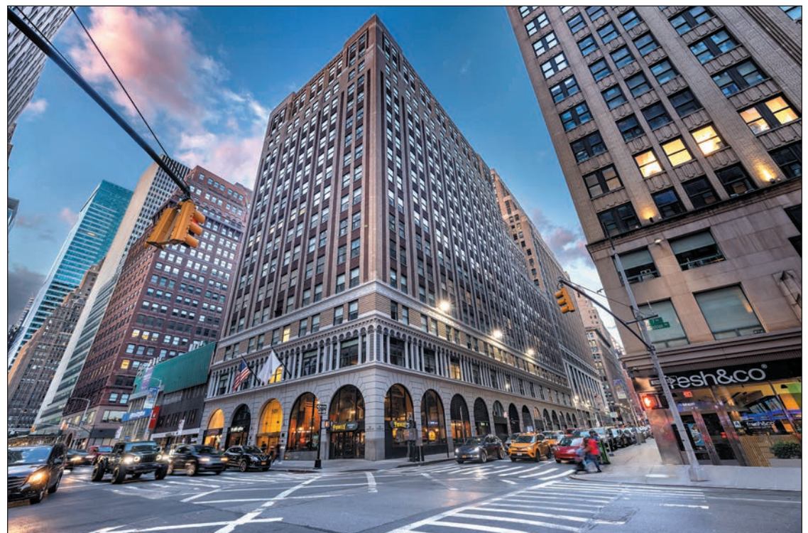
Located steps from Penn Station, 501 Seventh Avenue comprises 18 stories of modern office space for tenants
