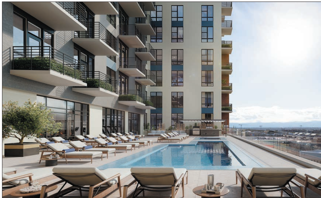
Rockefeller Group recently completed Patten Gray, its first luxury rental project in downtown Denver. The 250-unit project, located in Denver’s Golden Triangle neighborhood, prioritizes ample living space and amenities, and boasts 360-degree views of the Rocky Mountains
