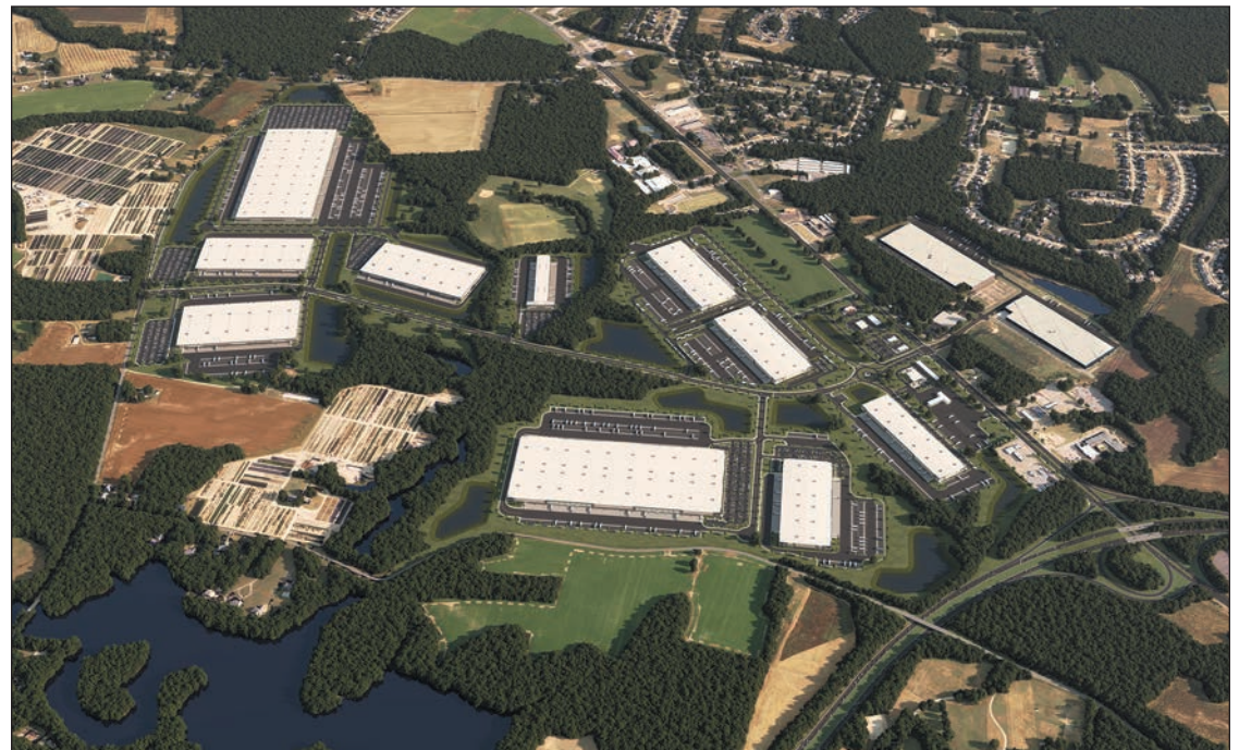
Rockefeller Group, in partnership with the Matan Companies, started construction in 2024 on Port 460 Logistics Center, a massive 5-million-square-foot industrial development project on 500 acres near the Port of Virginia
