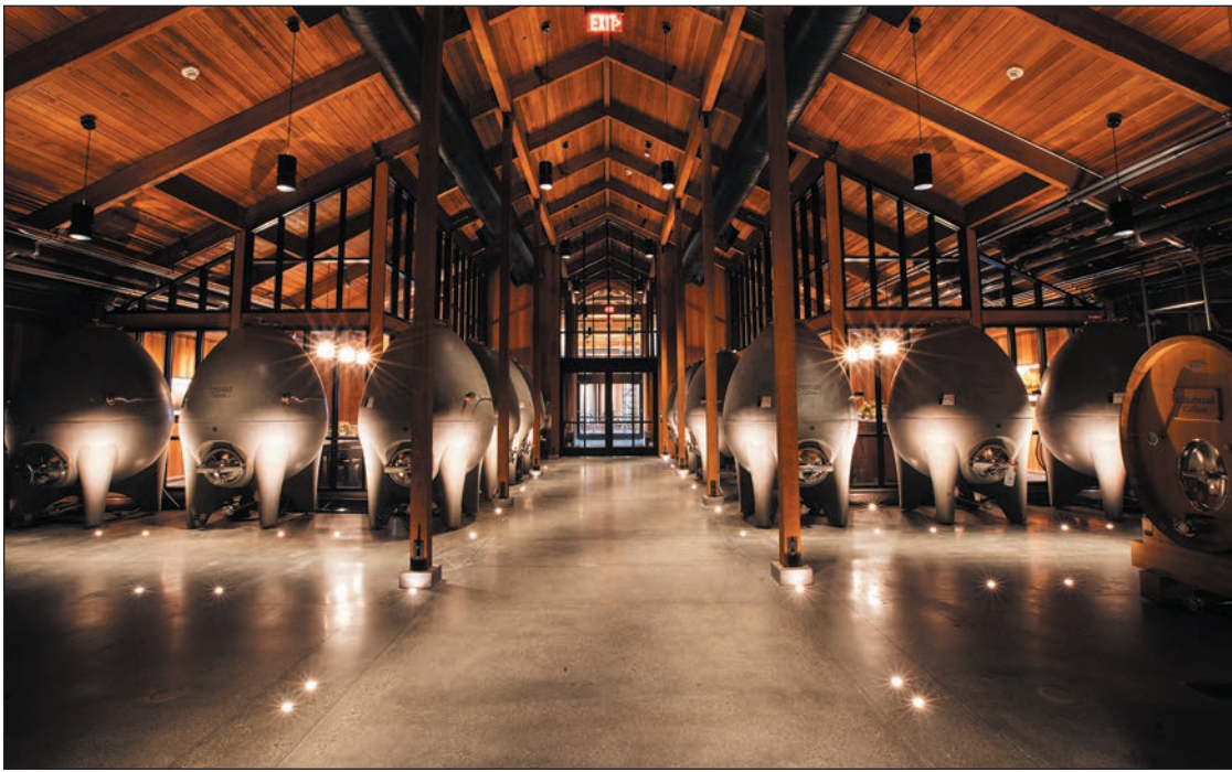
Cakebread Cellars uses concrete egg-shaped fermentation tanks in their fermentation hall
